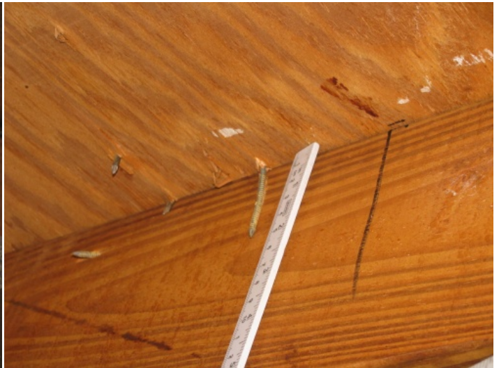
Roof Deck Attachment - 8d nails
