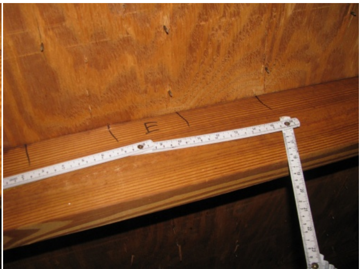
Roof Deck Attachment - 6" spacing in the field
