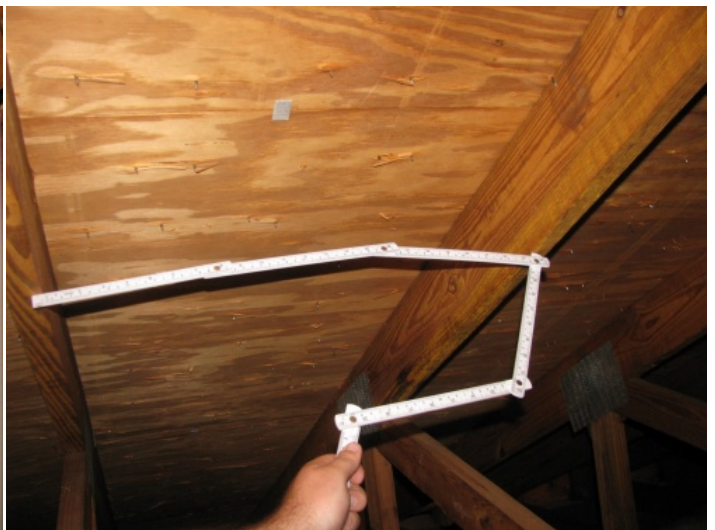
Roof Truss Spacing - 24"
