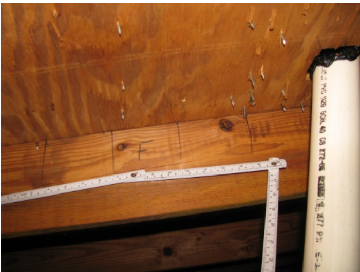
Roof Deck Attachment - 6" spacing in the field
