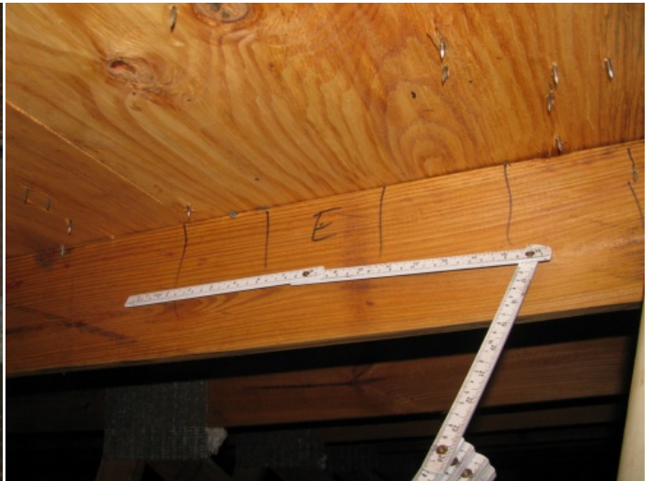
Roof Deck Attachment - 6" spacing on the edge
