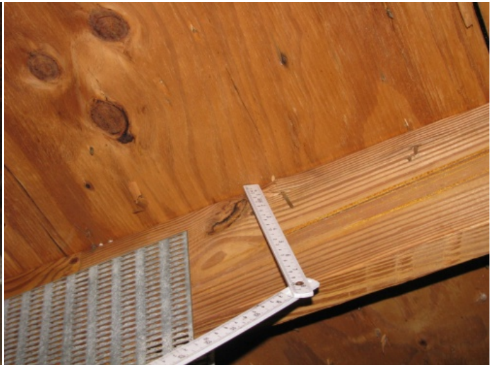
Roof Deck Attachment - 8d nails
