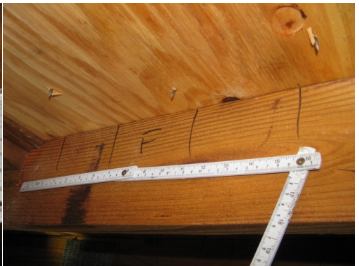
Roof Deck Attachment - 6" spacing in the field
