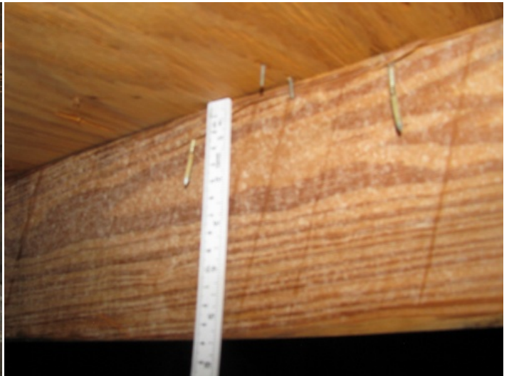
Roof Deck Attachment - 8d nails
