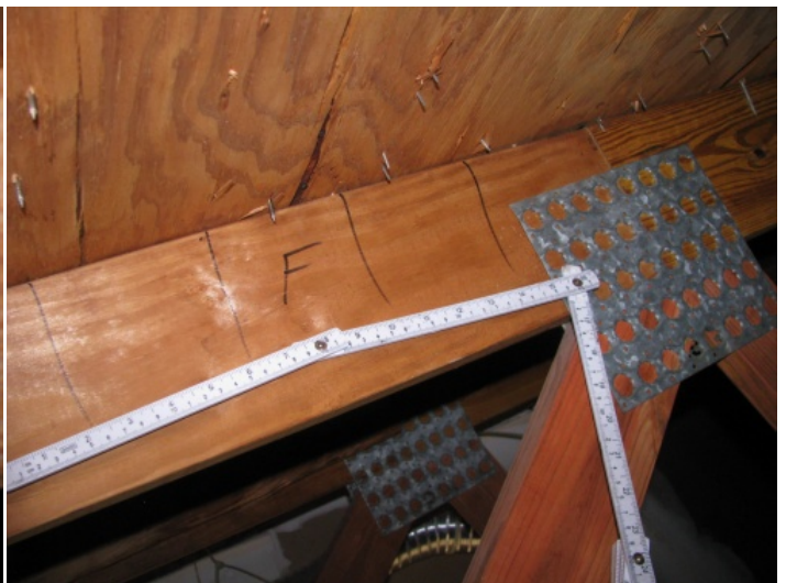
Roof Deck Attachment - 6" spacing in the field
