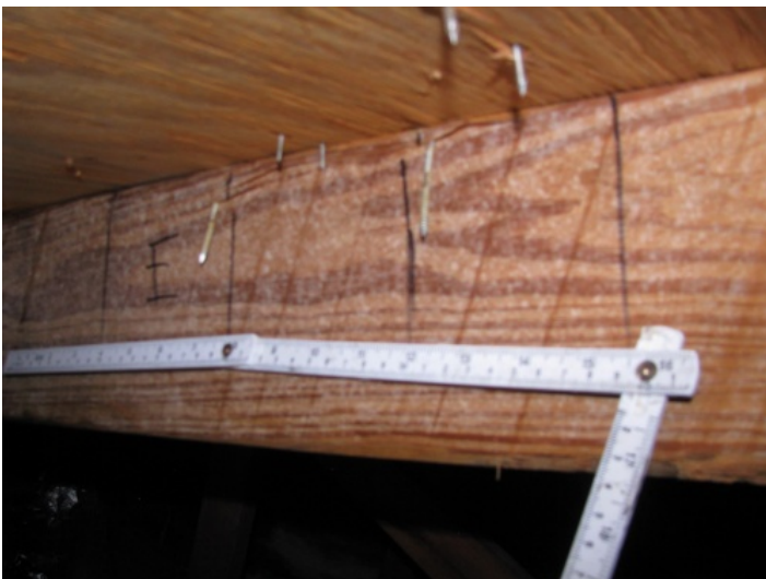
Roof Deck Attachment - 6" spacing on the edge
