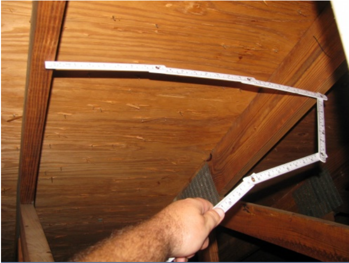
Roof Truss Spacing - 24"
