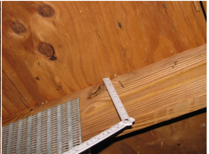
Roof Deck Attachment - 8d nails
