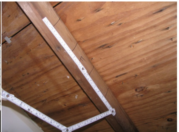
Roof Deck Attachment - 6" spacing in the field
