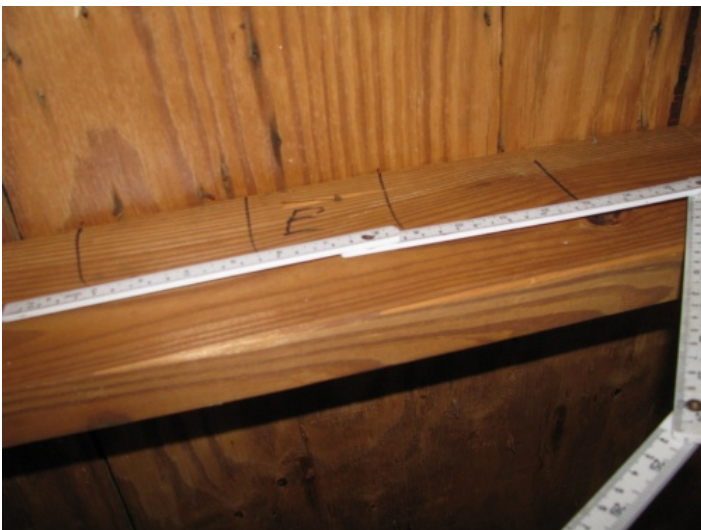
Roof Deck Attachment - 6" spacing on the edge
