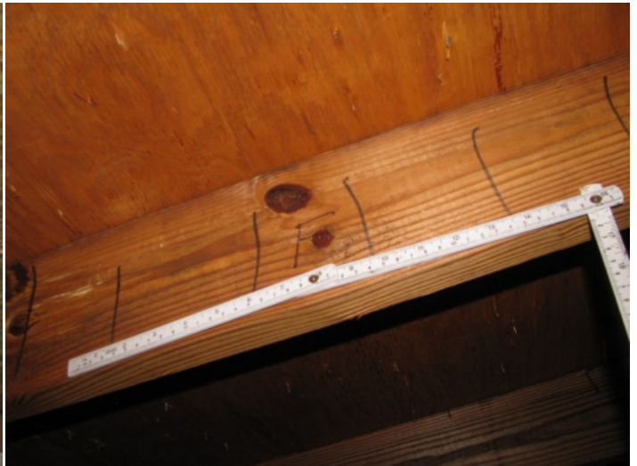
Roof Deck Attachment - 6" spacing on the edge
