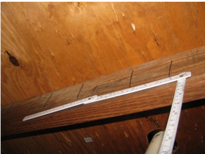
Roof Deck Attachment - 6" spacing in the field
