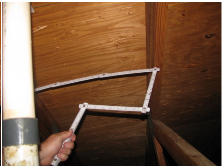
Roof Truss Spacing - 24"
