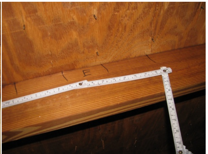
Roof Deck Attachment - 6" spacing in the field
