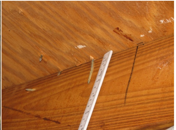
Roof Deck Attachment - 8d nails
