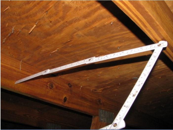
Roof Truss Spacing - 24"
