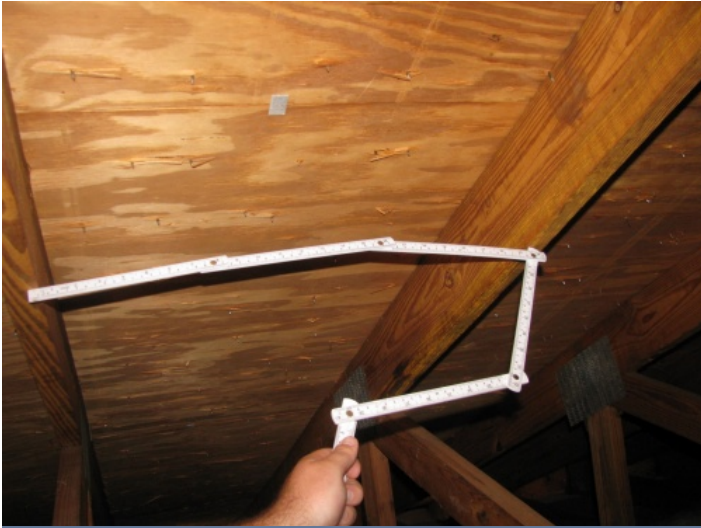
Roof Truss Spacing - 24"
