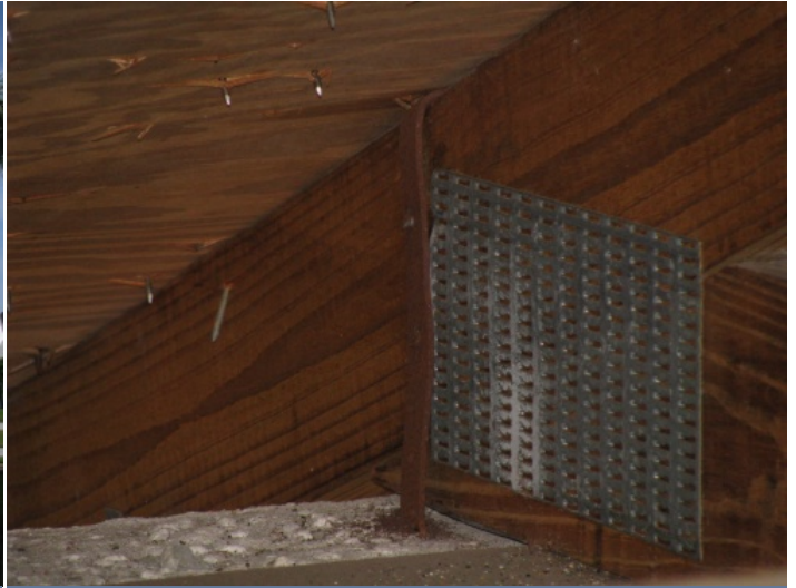
Roof to Wall Connection - single wrap straps front side with 2 nails
