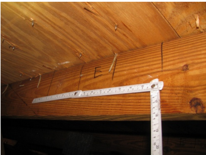
Roof Deck Attachment - 6" spacing on the edge
