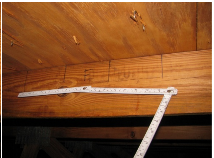
Roof Deck Attachment - 6" spacing in the field
