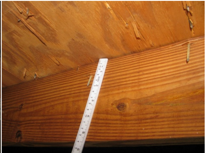
Roof Deck Attachment - 8d nails
