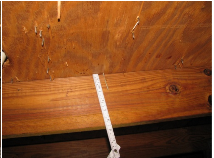
Roof Deck Attachment - 8d nails
