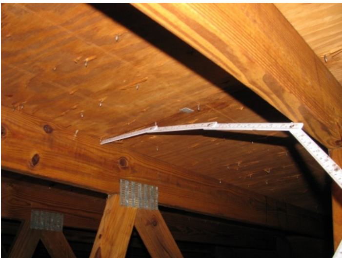
Roof Truss Spacing - 24"
