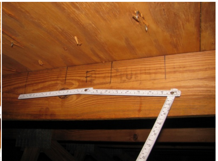
Roof Deck Attachment - 6" spacing on the edge
