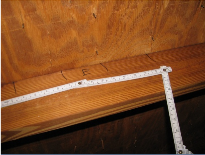
Roof Deck Attachment - 6" spacing in the field
