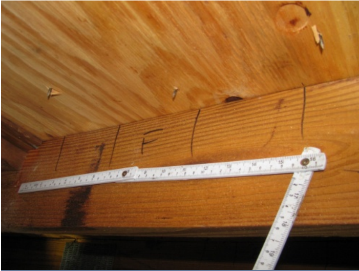
Roof Deck Attachment - 6" spacing in the field
