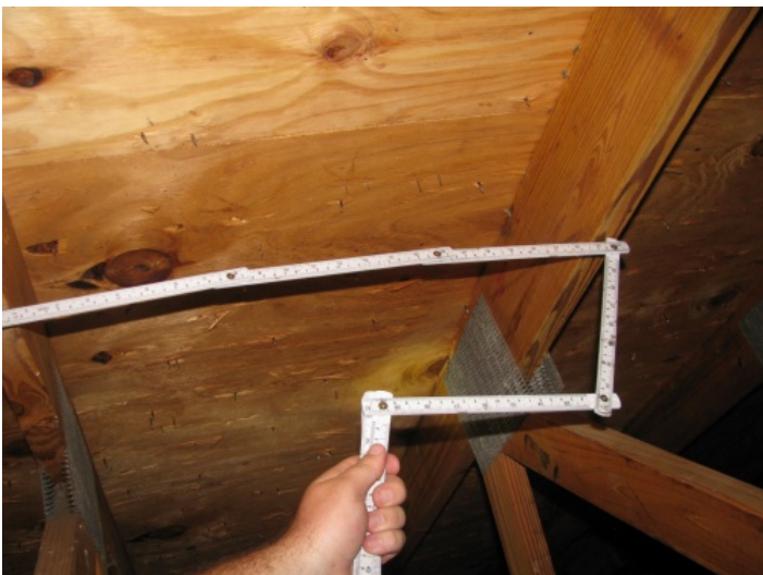
Roof Truss Spacing - 24"
