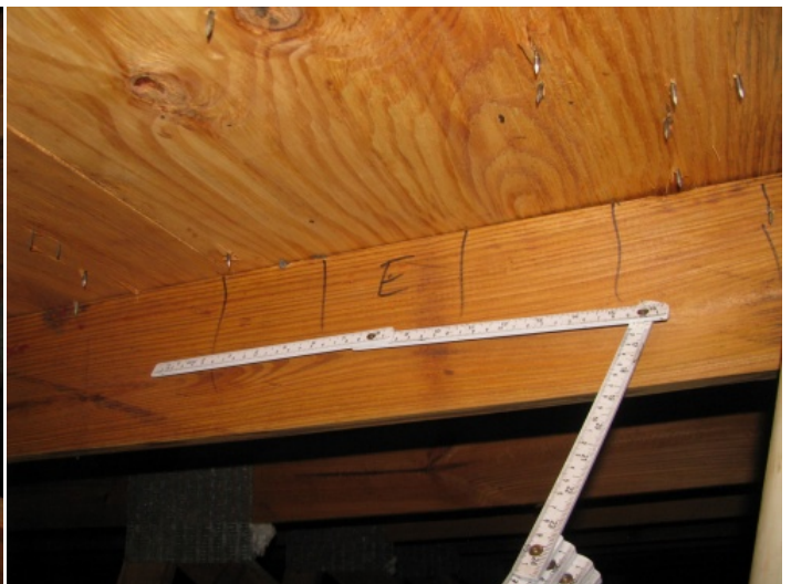
Roof Deck Attachment - 6" spacing on the edge
