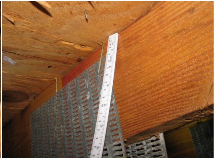
Roof Deck Attachment - 8d nails
